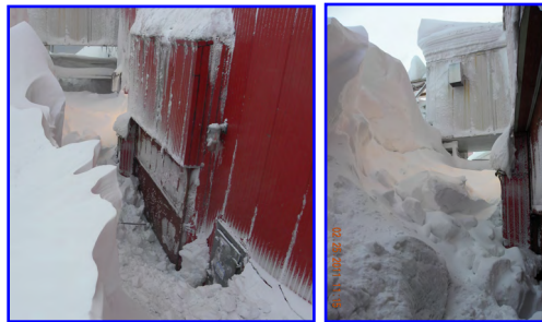
Snow drift blocking the 12 foot high M4A mill building garage door and man door.
